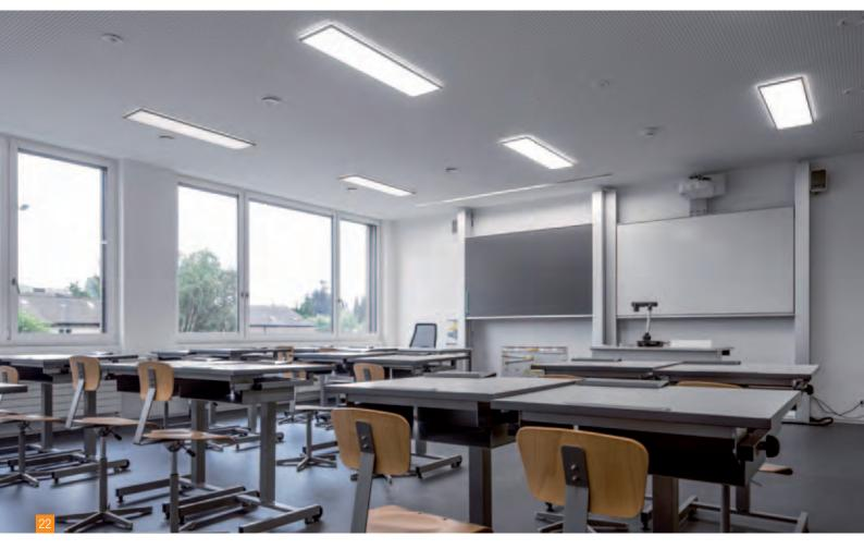
[22] Three ceiling-mounted rows of lights arranged parallel to the window façade provide homogeneous and glare-free light. (Photo: licht.de/Trilux)
