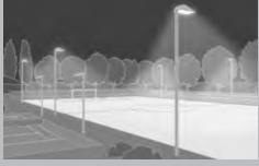
**Floodlights** on appropriately high masts are used for the efficient and homogeneous illumination of outdoor sports fields and other large areas.
