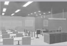
The fixtures of **recessed luminaires** are flush-mounted in the ceiling, wall or floor. Accordingly, only the light itself can be seen, with the housing of the luminaire becoming practically invisible.
