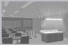
**Pendant luminaires** are mounted at a distance below the ceiling and serve as design elements in a room. They provide direct/indirect light distribution and come in a wide variety of designs.
