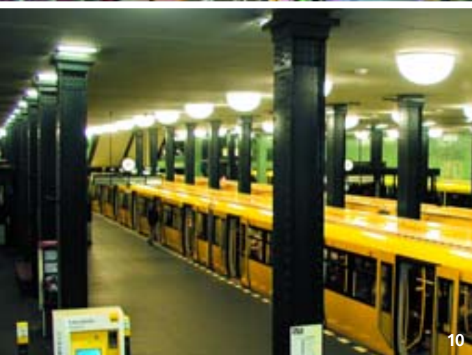
Ring-shaped induction lamps in use: manufacturing bay (Photo 9), Alexanderplatz underground station in Berlin (Photo 10), high-bay warehouse (Photo 11), library (Photo 12), works entrance check-point (Photo 13), car showroom (Photo 14).
