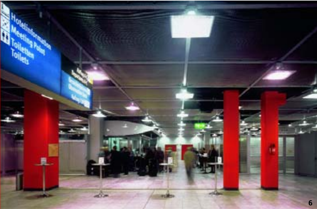
Photo 6: Maintained lighting in an airport building, a typical application for induction lighting.
