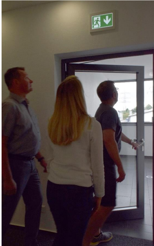
Fig. 1 Existing door sign in escape and rescue routes. People escaping have clearly understood the meaning of the arrow above the door and reacted correctly. Source: Inotec
