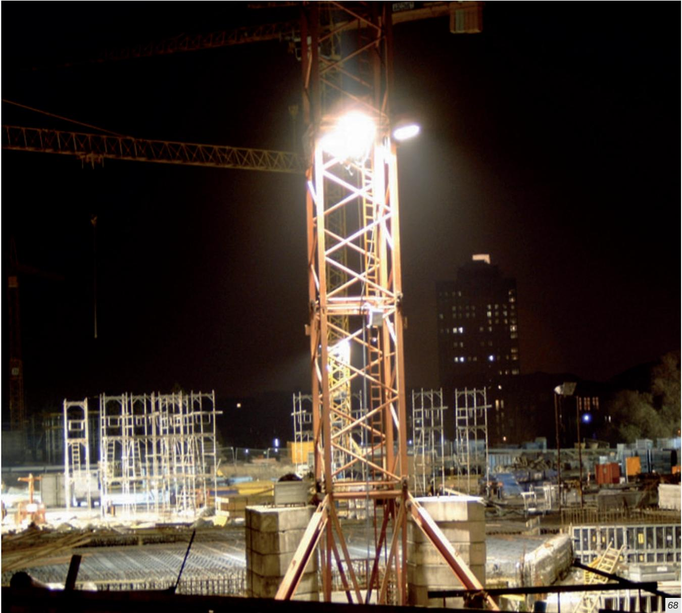
**Arrangement of luminaires:** Wherever possible, no luminaires should be positioned in the actual area where manpower and machines work. As work areas often change, mobile lighting – directed inwards from the perimeter – is useful. Generally speaking, in addition to the measures mentioned above, the mobility required can be achieved either with small mobile luminaires or with adjustable floods on high masts.
