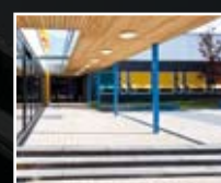
Schoolyard and park- ing facility lighting Page 42-43
