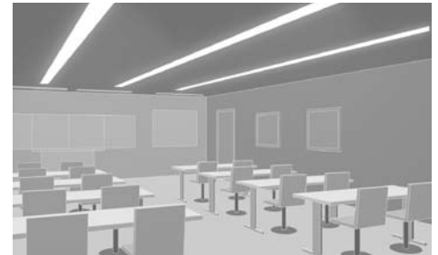
Continuous row systems (surface-mounted, recessed) for fluorescent lamps are rows of through-wired luminaires fitted with various anti-glare devices such as reflectors, louvers or prismatic enclosures.
