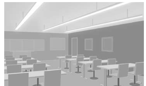
Continuous row systems (suspended) for fluorescent lamps are available with various enclosures (reflector, louver or prismatic). To give a greater sense of space, preference should be given to models with an indirect lighting component for illuminating the ceiling.
