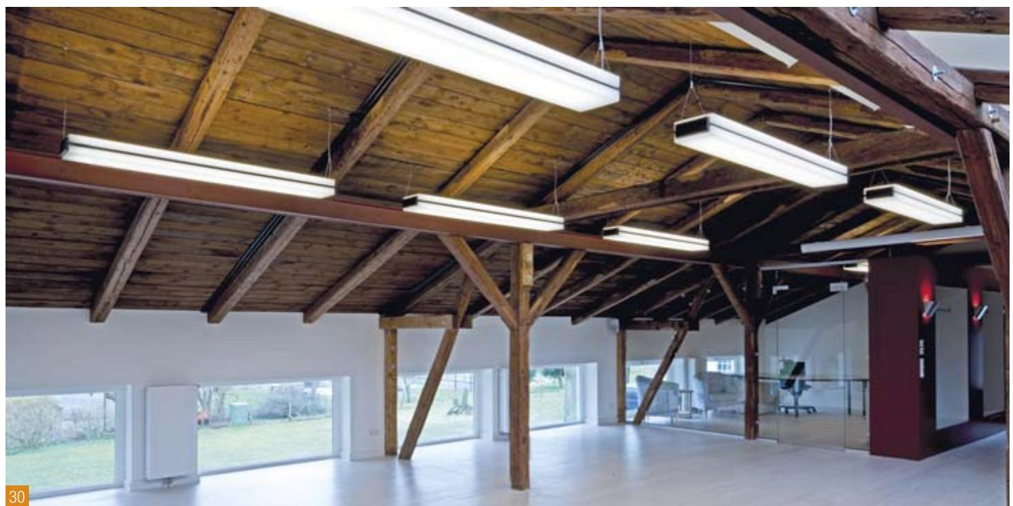
ation when they are not needed. Daylight sensors allow artificial lighting to be regulated according to the amount of natural incident light available. Constant light regulation – the so-called maintenance feature – dims luminaires to the maintained illuminance required and thus saves energy.
