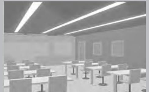
**Continuous-row systems (surface-mounted or recessed)** are series-connected and trunking luminaires that are equipped with different optics and anti-glare devices.
